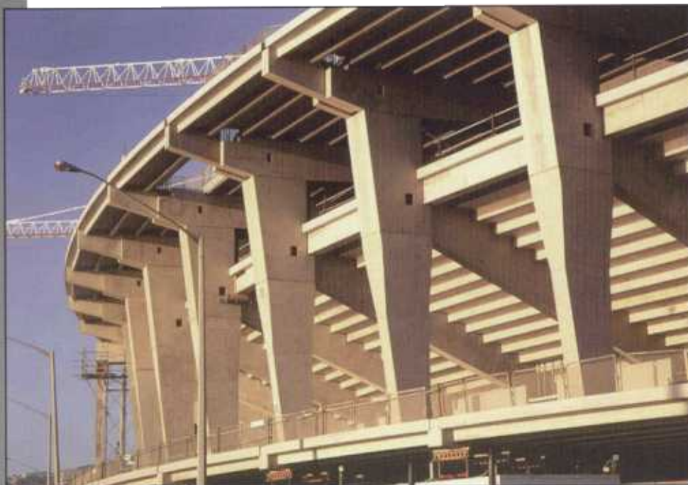
Exterior of 40,000-seat Wellington Stadium nearing completion
