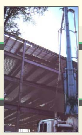
Pumping Structural Lightweight Concrete on Steel-Frame Construction
