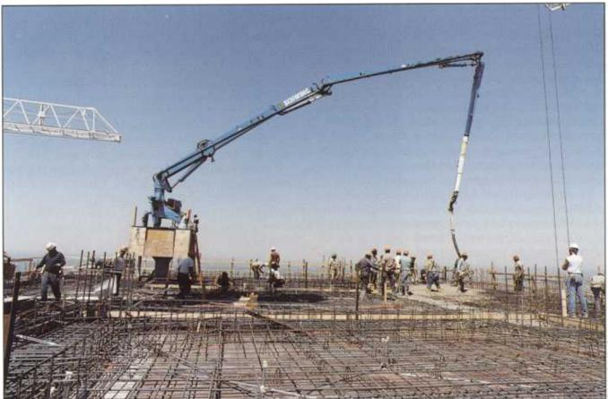
Lightweight concrete was pumped up to 760 feet to construct the 800-foot-high mixed occupancy building at 900 N. Michigan Ave., Chicago. On some buildings, lightweight concrete has been pumped more than 1,000 vertical feet. Protruding rebar is a serious safety concern; see page 589 for more information on reinforcing steel safety.
