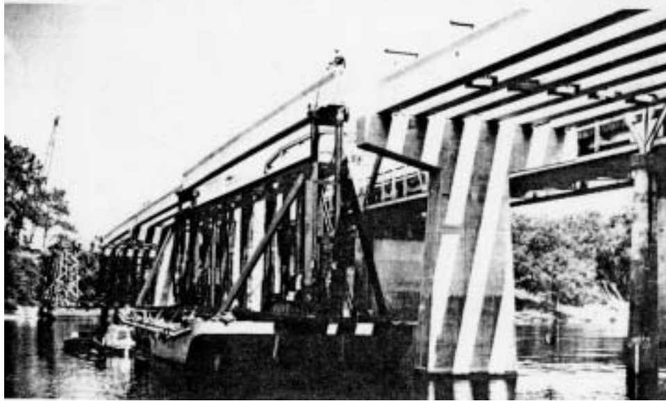
Figure 16. Barge-mounted frame placed beams (to the right is an old truss bridge; both bridges will carry U.S. 19 traffic) (Brown, Larsen, and Holm 1995)
