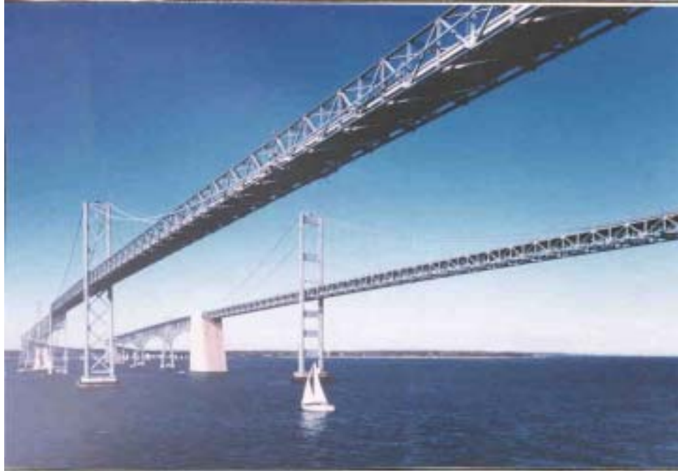
Figure 27. Chesapeake Bay Bridges, Annapolis, MD
