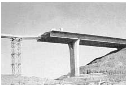
Figure 1 Napa River Bridge during construction.
