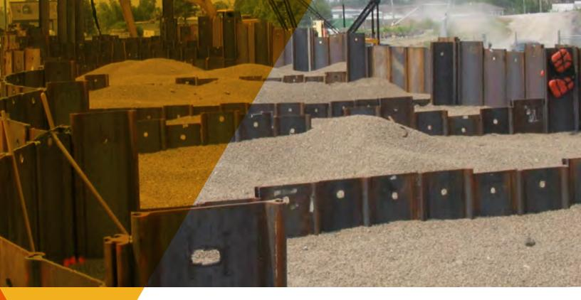
As less buildable land is available, the need for creative solutions for today's unique geotechnical challenges becomes obvious. Soft and unstable soils along with tight construction schedules are common in several areas of the country. The use of compacted fills utilizing Expanded Shale, Clay and Slate (ESCS) lightweight aggregates is a proven solution for these problems.
