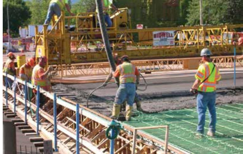
Figure 5. Internally cured concrete being placed on the Court Street Bridge in Syracuse, New York.
