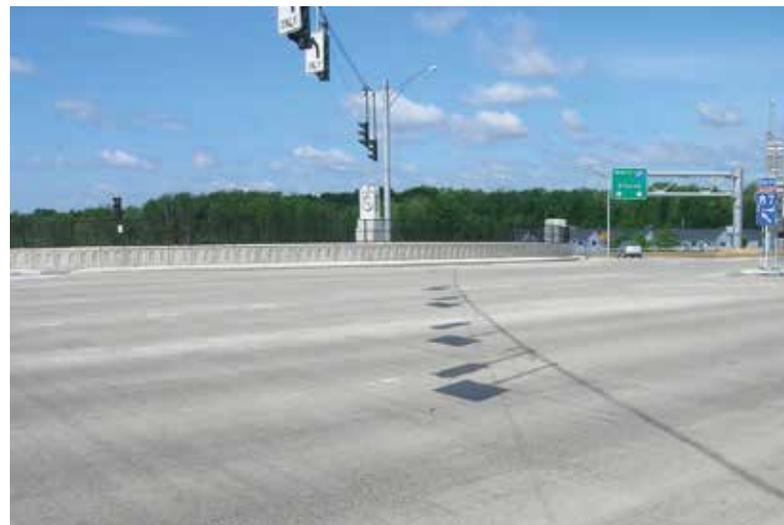
Figure 4. SPUI Bridge deck utilizing lightweight concrete to reduce cracking.
