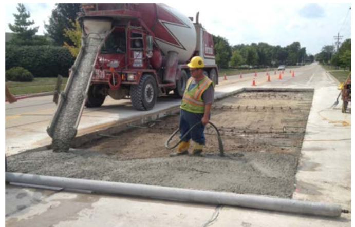
Figure 3. Internally cured mixtures being used for panel replacement.
