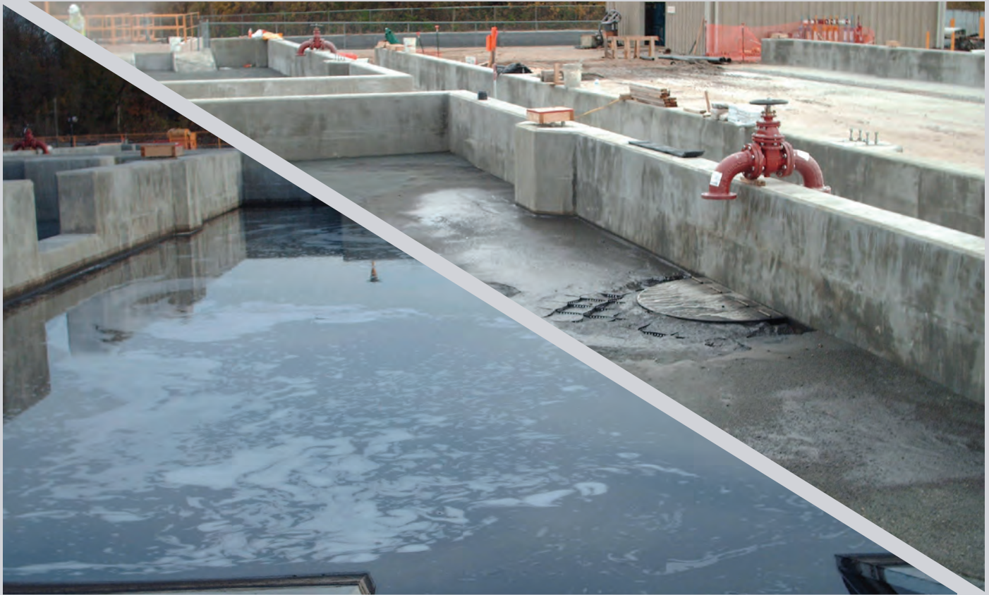
Industrial Sludge Bed Media
