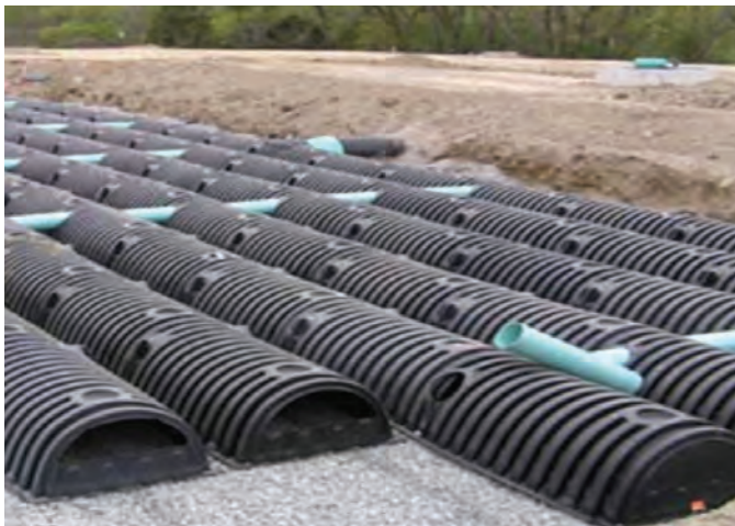
Storm Water Bed Filtration
