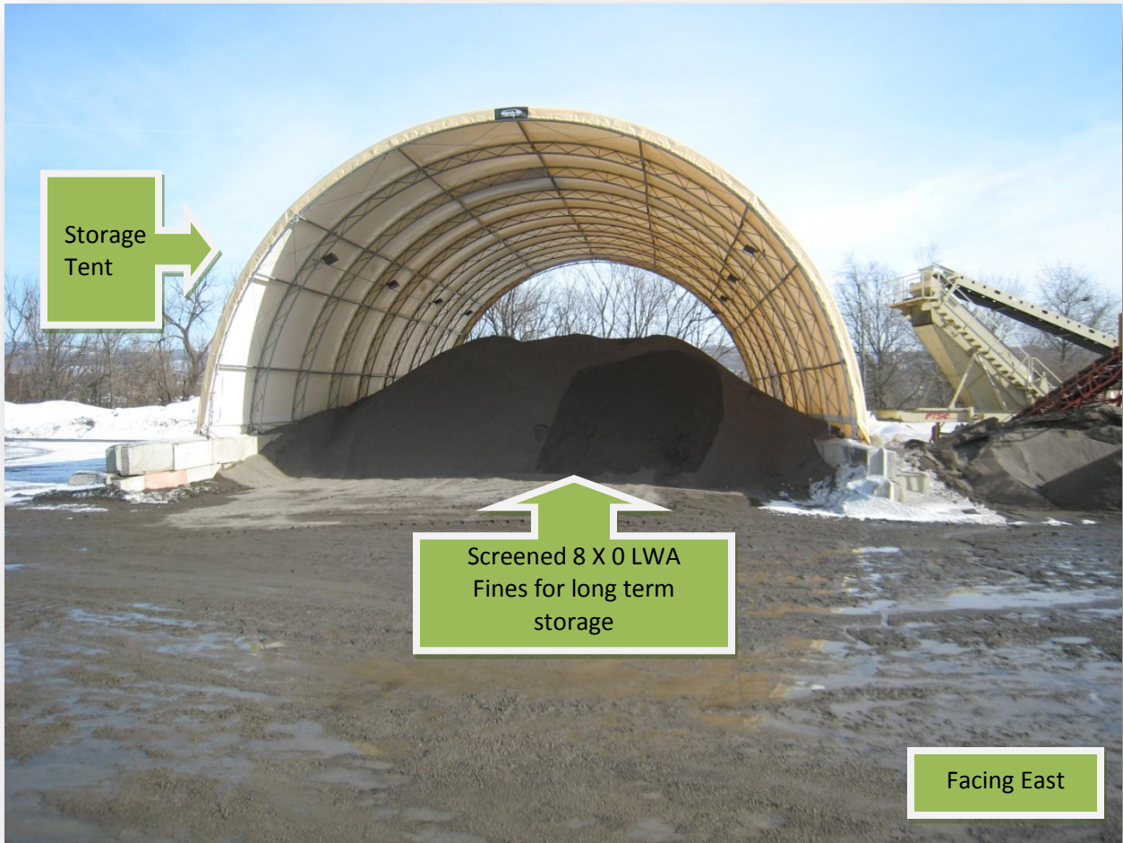
Figure 5. 8 X 0 LWA Fines storage tent. The tent allows for up to two weeks of storage of material. The increased covered storage allows the Fines Processing Area to be shutdown during unfavorable wind conditions.
